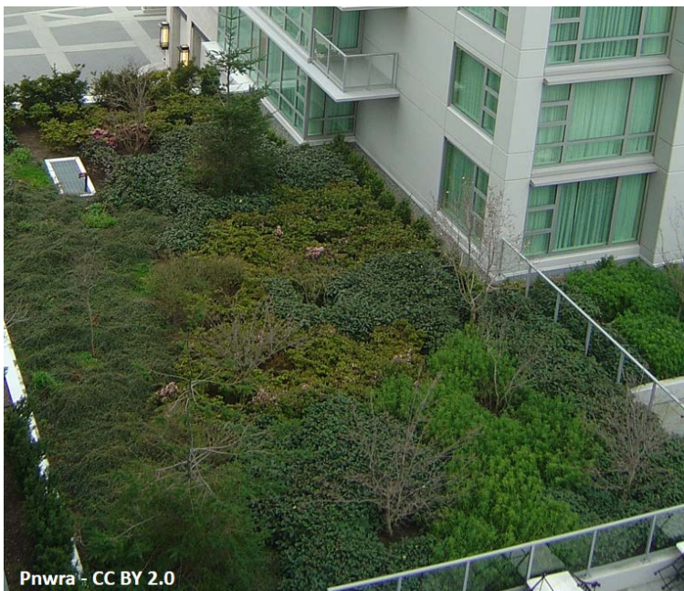
Figure 6: Green roofs not only counteract the urban heat island, but also increase the energy efficiency of buildings.
