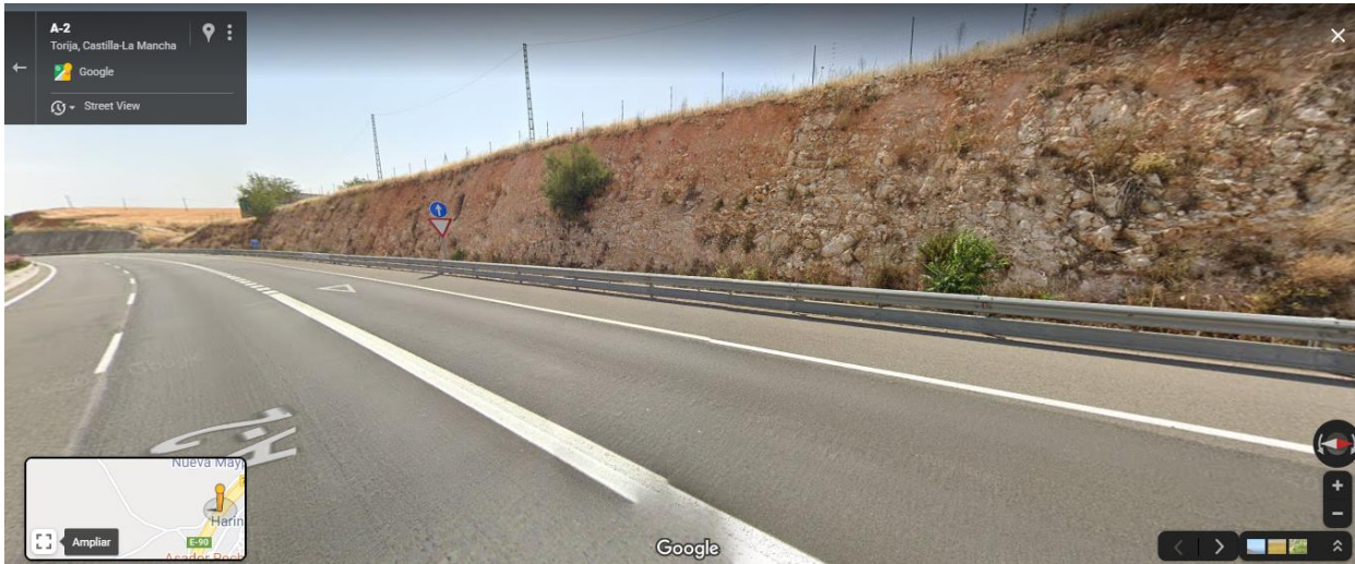
Figure 82: Side view of slope at pk 72+900 to pk 73+150
